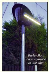
Light, has net zero carbon emissions, illuminates 16m of pathway and operates on a body temperature motion sensor to conserve energy and increase
